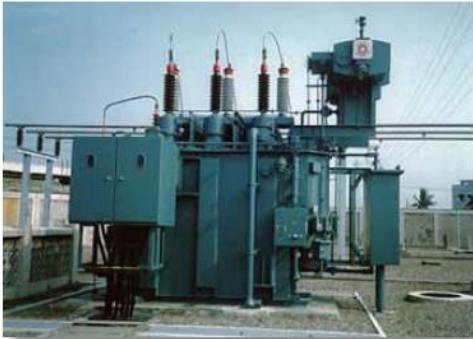
Low Noise Type Transformer 69kV-25MVA (50dB)
